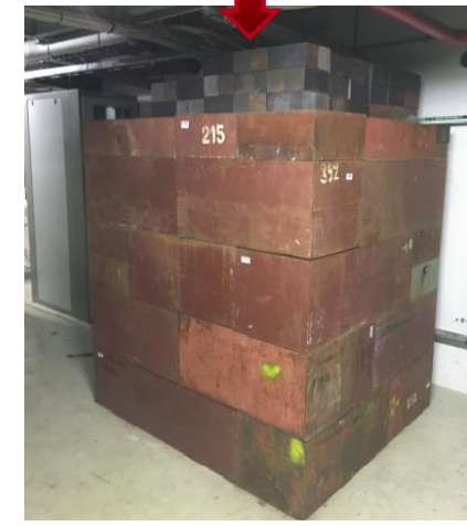
Shielding wall for the SPS access system
